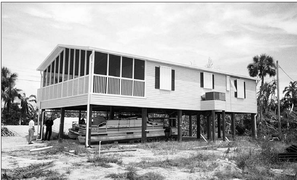
Figure 8-4. Manufactured home on a pile foundation.
