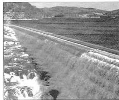
Figure 17 Though still meeting safe drinking water standards, some of New York City's 19 reservoirs have been adversely impacted by runoff and other non-point source pollution in recent years. Protecting floodplain resources throughout the watershed, such as by preserving and restoring vegetated riparian buffers, will help to maintain and enhance the drinking water for over 9 million people.
