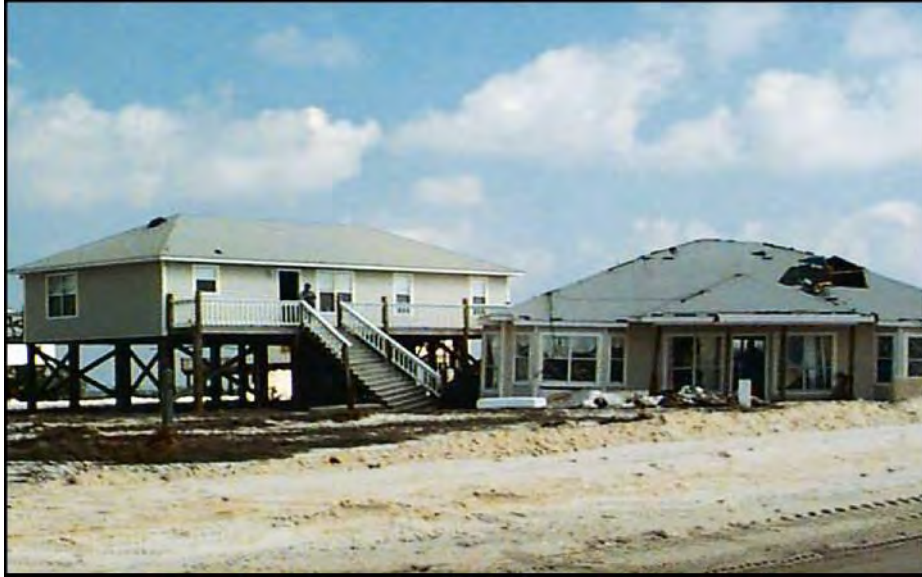
Figure 19. Hurricane Georges (1998), Dauphin Island, AL. As a result of erosion, scour, and inadequate pile embedment, the house on the right was washed off its foundation and into the house on the left.
