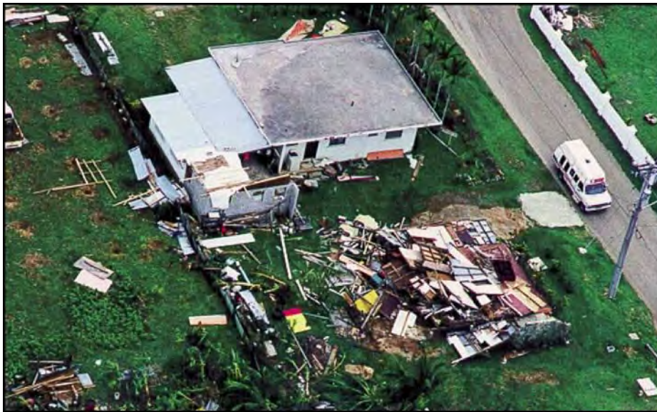
Figure 31. Typhoon Paka (1997). Although damaged by the storm, the concrete house in the upper part of the photograph survived, while the wood-frame house next to it was destroyed.
