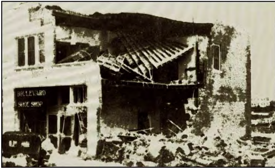
Figure 10. Building damage from 1926 hurricane, Miami, FL.
