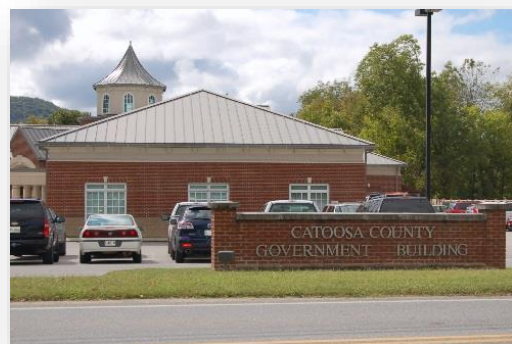
Figure 6. Catoosa County Government Building, Ringgold.
